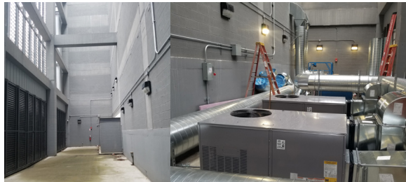
Before and after of UChicago Medicine corridor with commercial rooftop units
